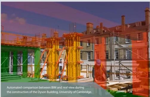
construction, the position of the camera can be tracked and the required 3D design information for the area under inspection will be automatically projected in his/her view.
